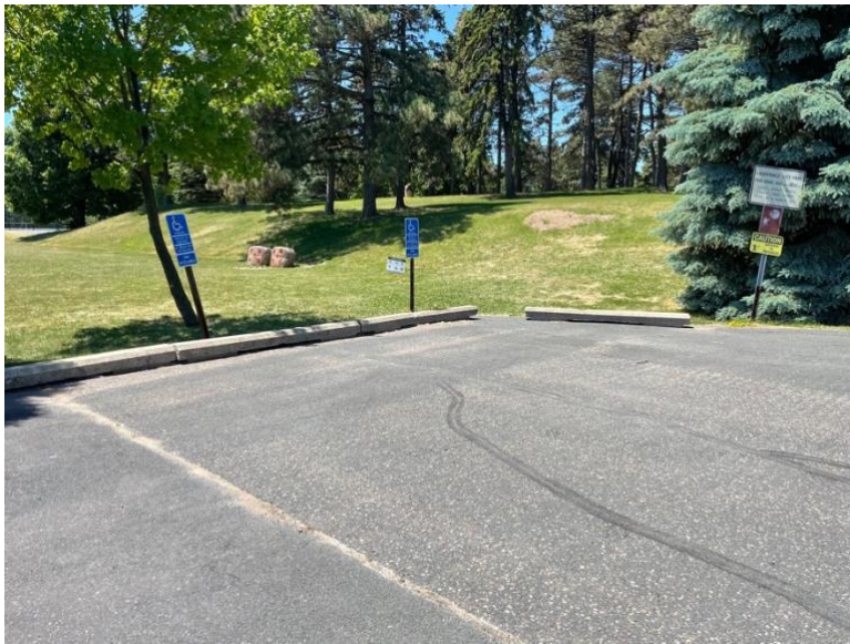
This photo shows an area with accessible signs but missing striping and a van access aisle.
