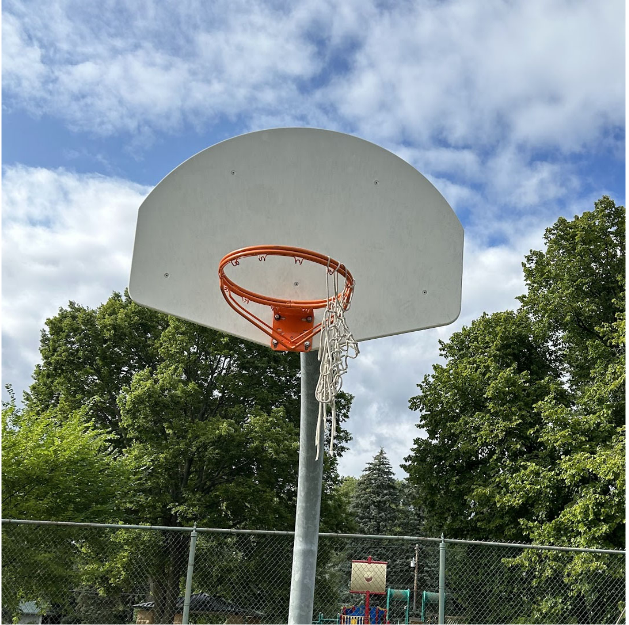
Backstop needs fencing repair.
