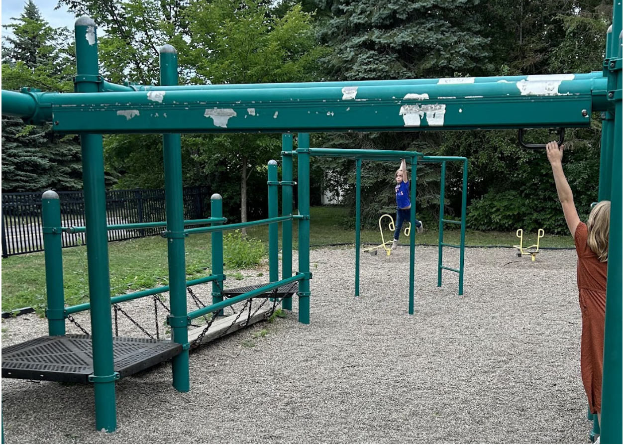
Chain ladder is broken on the bottom.
