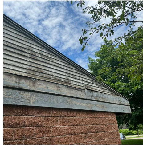
Southeast facade – Wood siding missing and paint flaking
