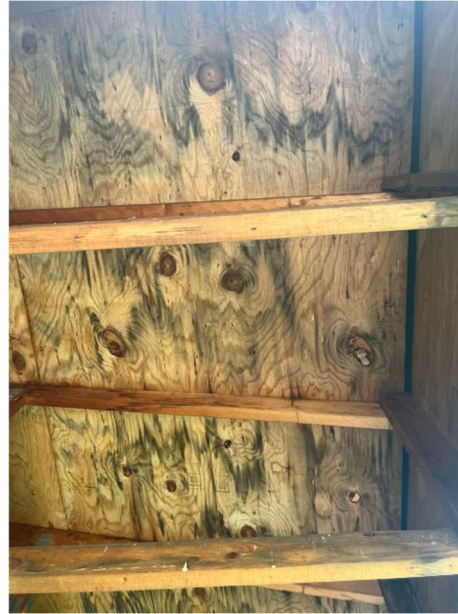
Missing soffit on north elevation – evidence of water damage
