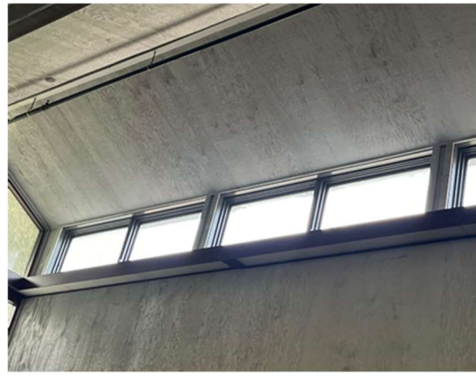
1982 Clearstory windows – seals broken, moisture and fog present
