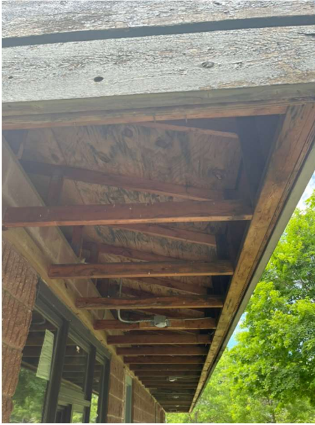
Missing soffit on north elevation – evidence of water damage
