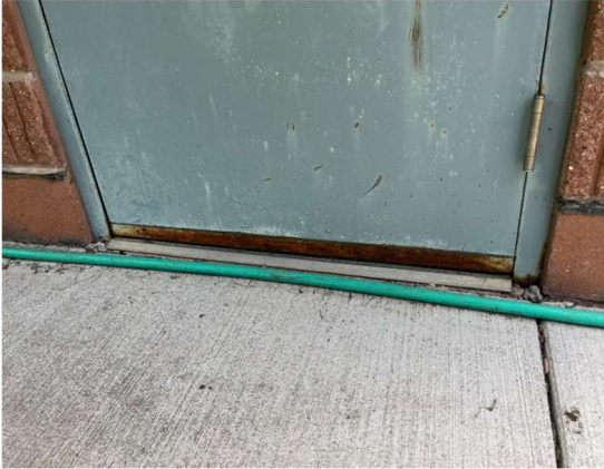
1982 original doors located on North elevation – rust damage
