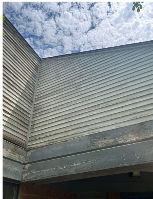
Southwest facade – Wood siding loose and paint flaking
