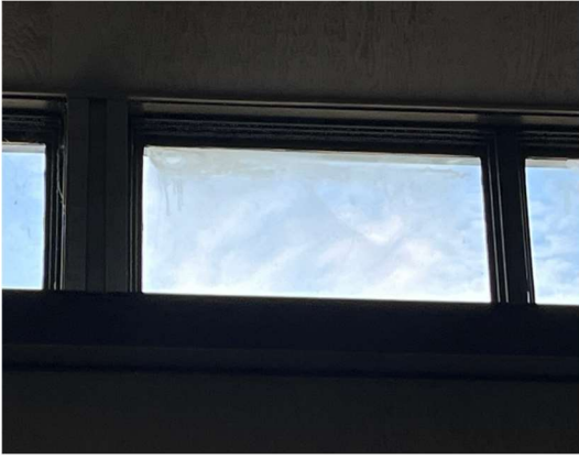
1982 Clearstory windows – seals broken, moisture and fog present
