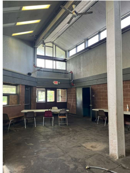
Interiors – multi-purpose room outdated finishes and showing signs of significant wear on the floors.
