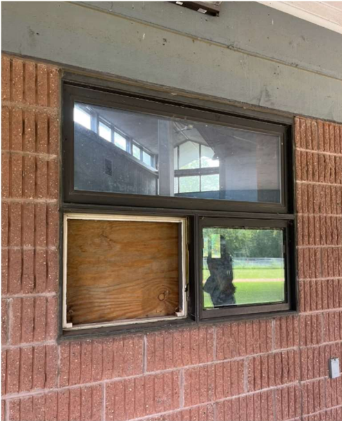
1982 original windows located on south elevation – broken pane and cracked seals
