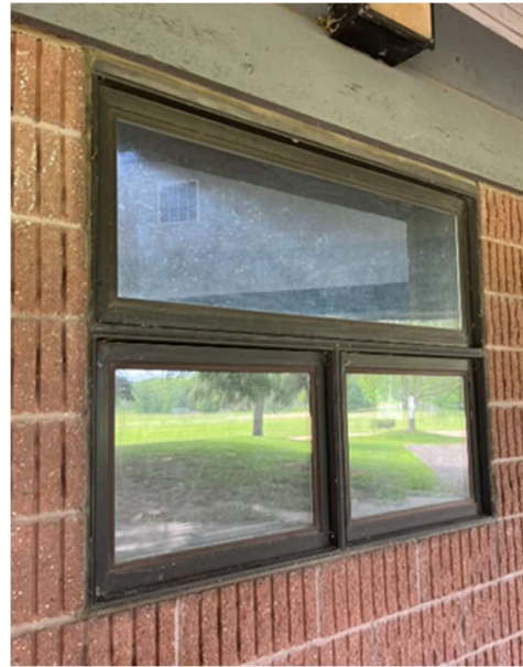
1982 original windows located on south elevation – broken pane and cracked seals
