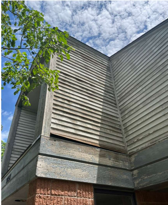
Southwest facade – Wood siding loose and paint flaking
